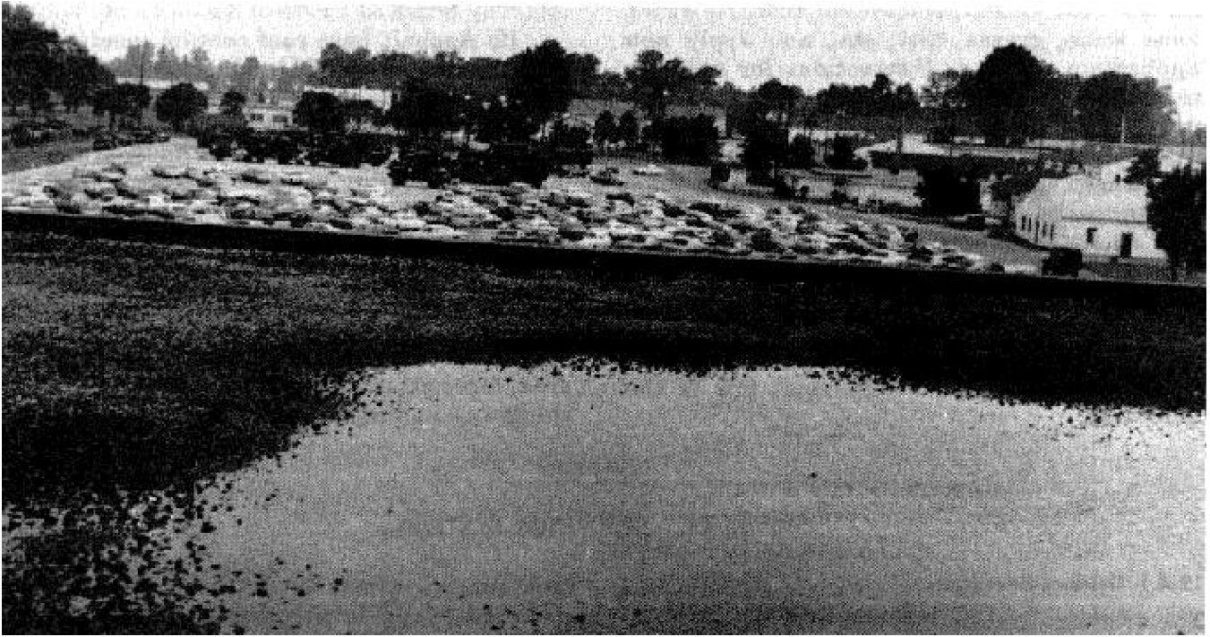
Figure 52. Drain not located in low area — ponding sometimes caused by structural defect.
