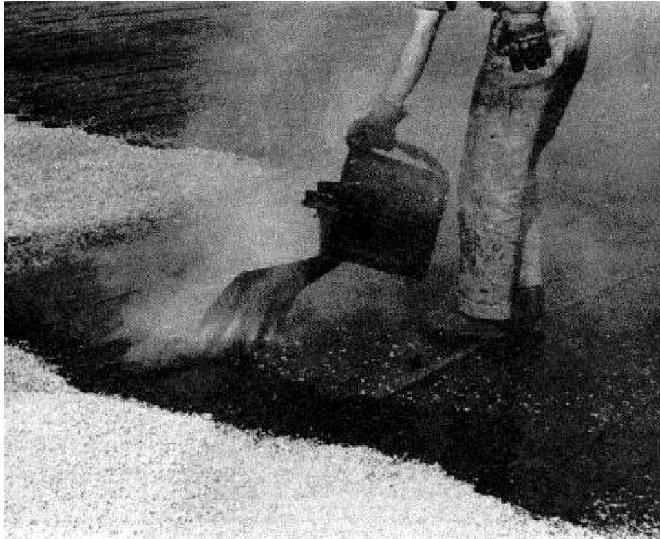
Figure 10. Surface coating of hot bitumen should be poured, not mopped.
